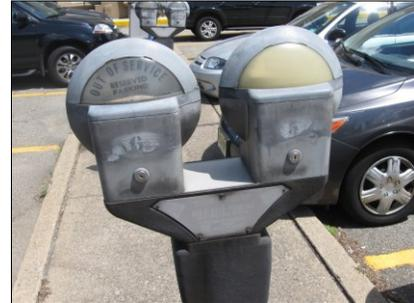
Some on and off-street meter housings are dual heads with a single vault and 1 coin canister. It is recommended that in high volume parking areas, the dual meter housings be replaced with single head housings mounted on a yoke that permits 2 single head meters to be installed on one meter pole to control two parking spaces.
